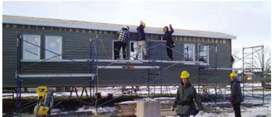
*ABOVE: Students work on soffits and roofing finishes, outside in -10°C!*
